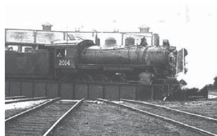
This turntable was used to rotate trains back onto the tracks after servicing
